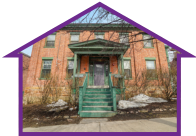
Main Street Family Shelter
