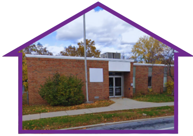
Warming Station and Future Waystation Shelter
